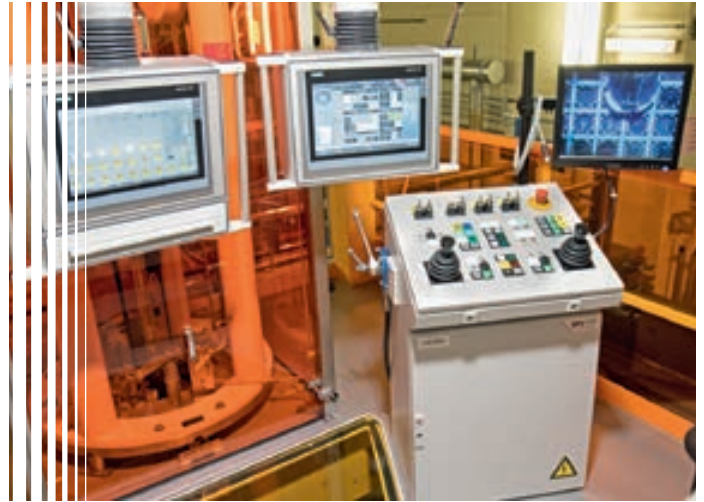
Operating platform after refurbishment of the refueling machine
