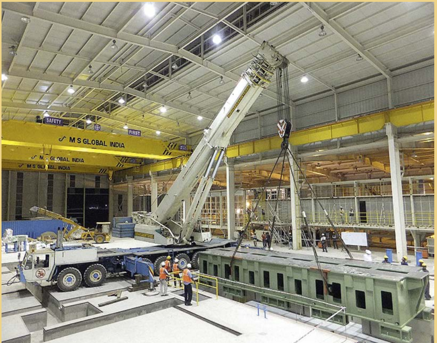
Installation of the lower beam
