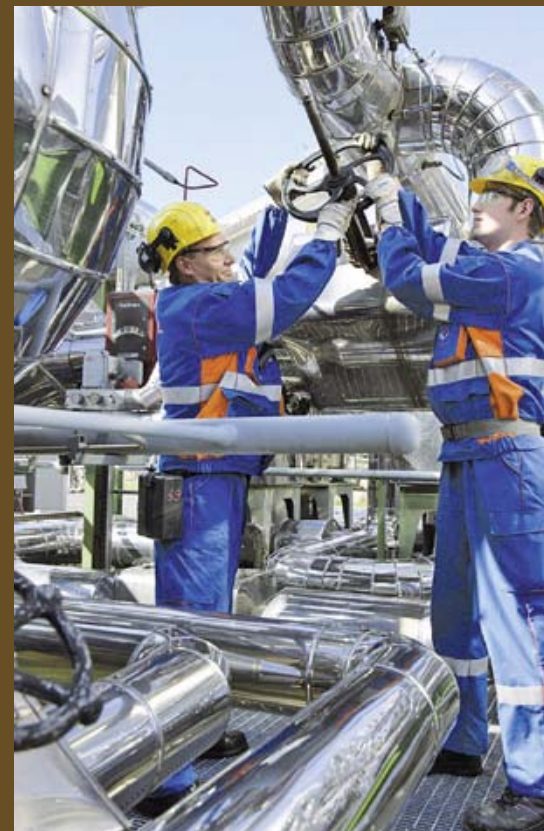
Repair of valves
