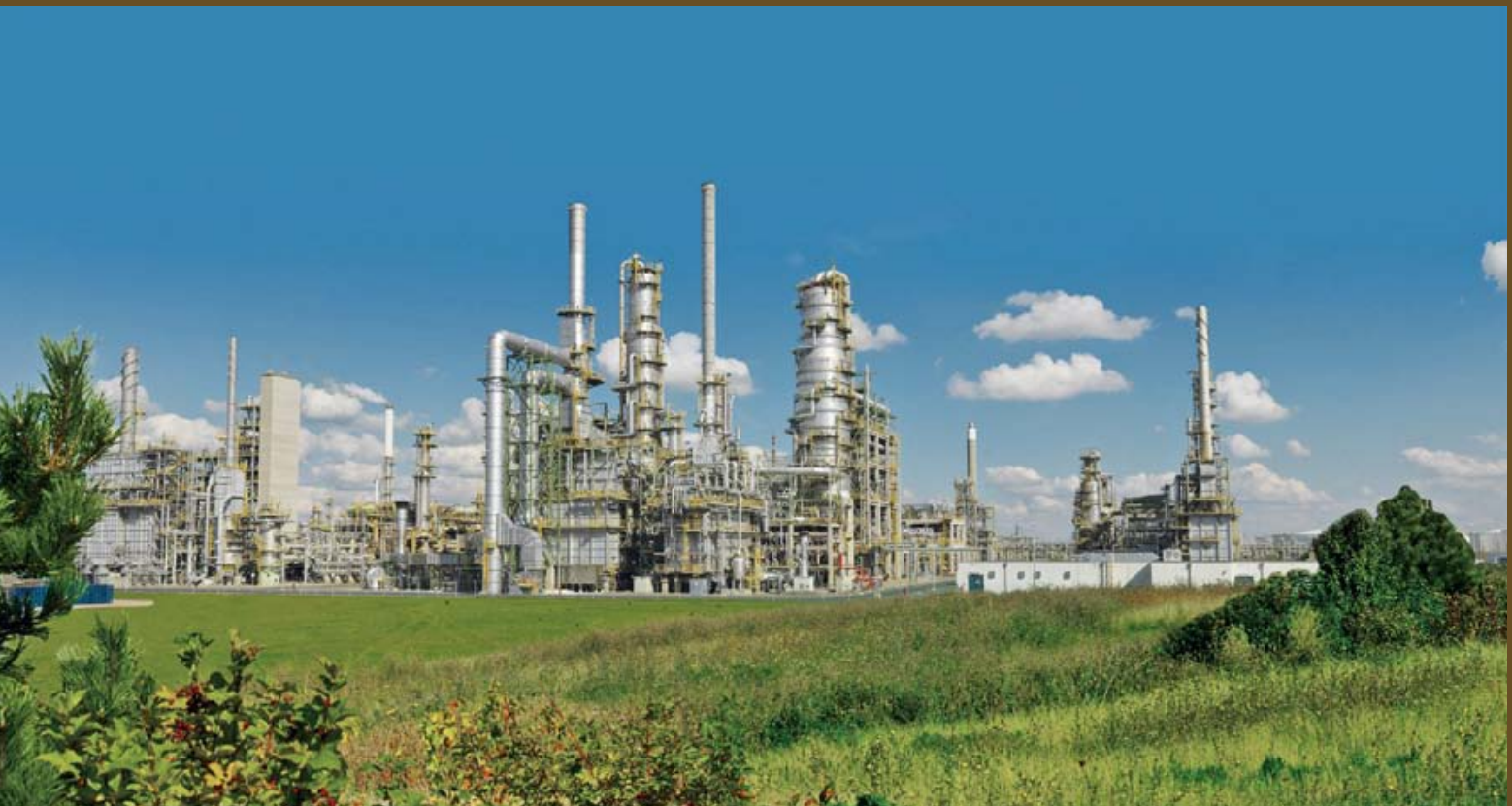
The TOTAL refinery connected to power – © Matthias Kuch
