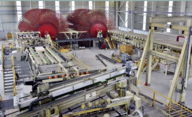
Cooling and stacking line during installation
