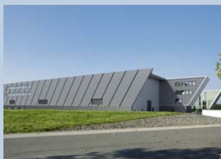
OHLF building, south view
