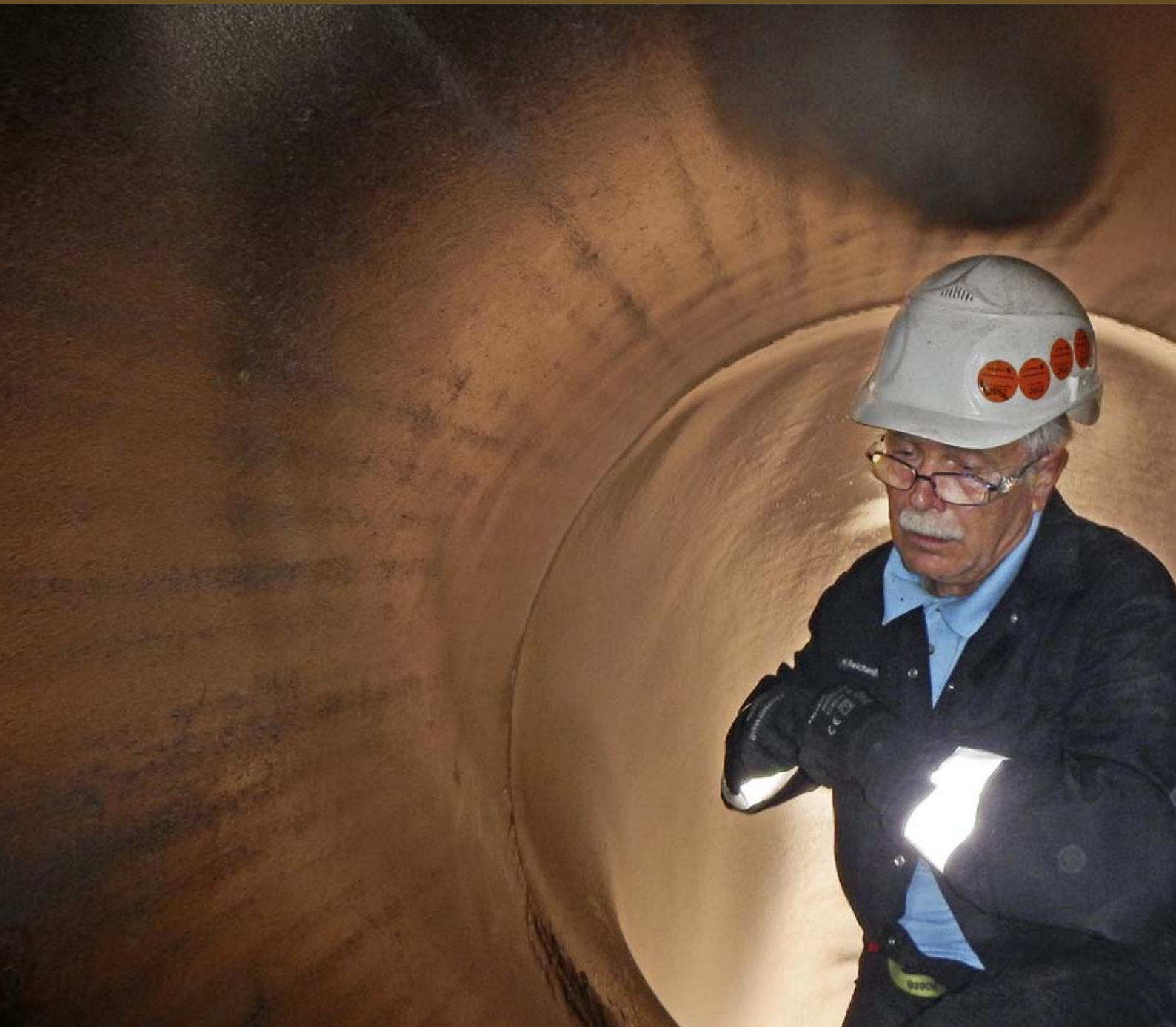
Visual checks in a piping section
