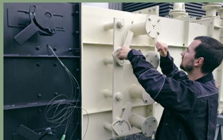
Outside the new burner duct, preparations are made for the next series of tests
