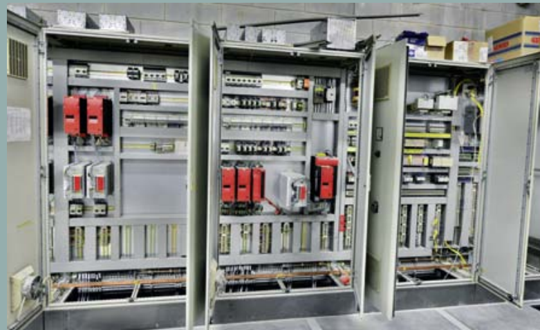
Electrical system upgrade
