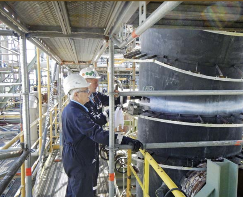
Ultrasonic testing on a weld seam
