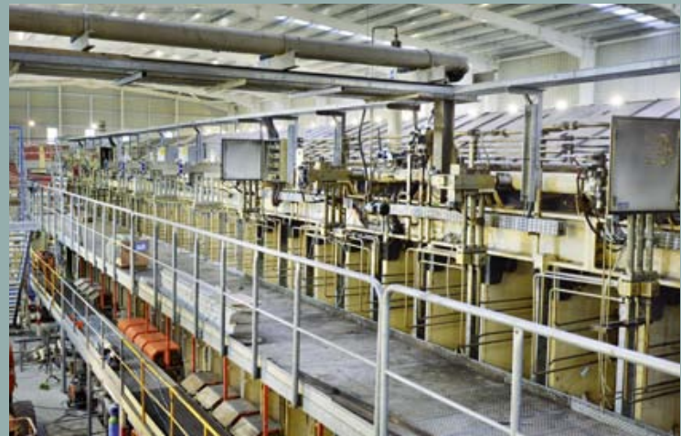
Partially rebuilt hydraulics
