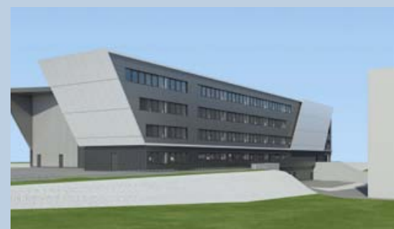
OHLF building, north view
