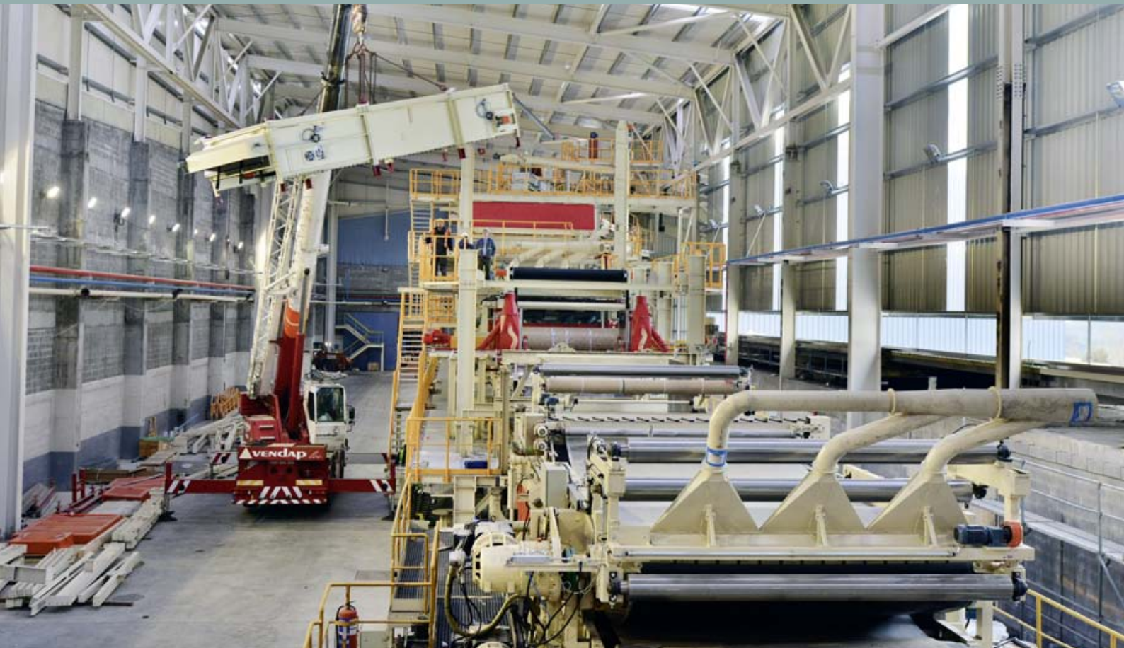
Installation of mat former bunker
