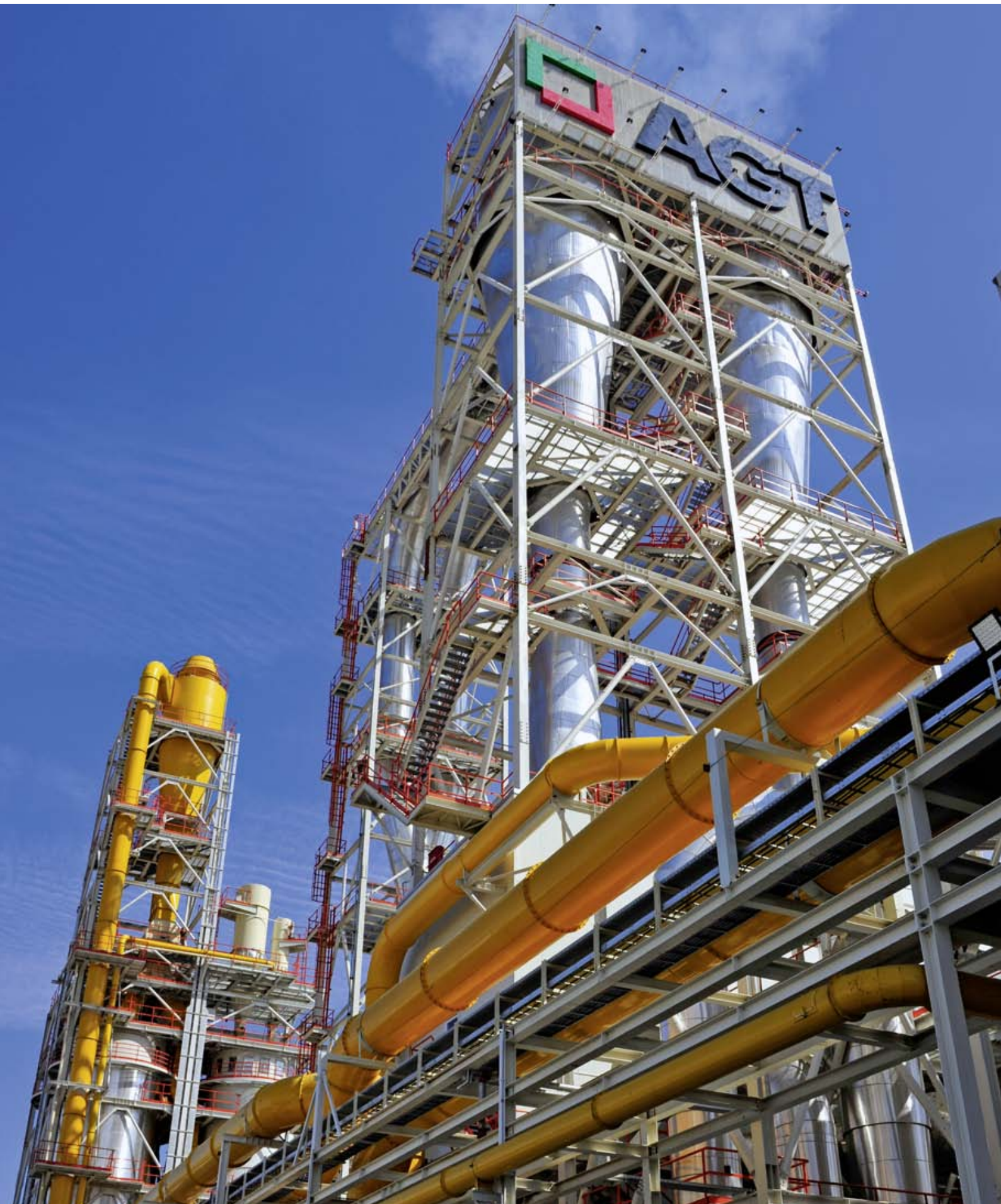
The new MDF plant at AGT, Antalya, Turkey
