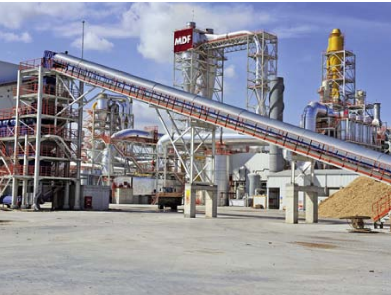
Energy plant and MDF dryer
