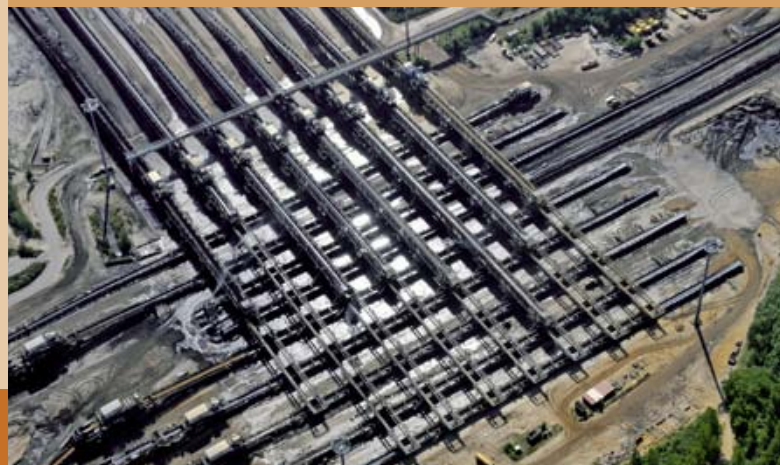
RWE belt transfer point
