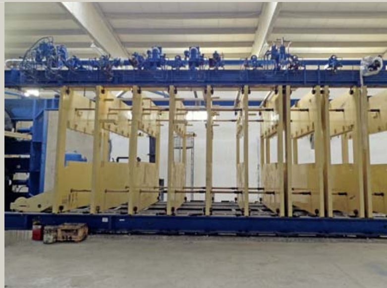
Installation of the frames for the ContiRoll®
