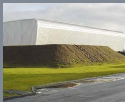
Magnox interim storage facility in Berkeley, with a storage capacity of up to 1,004 containers
