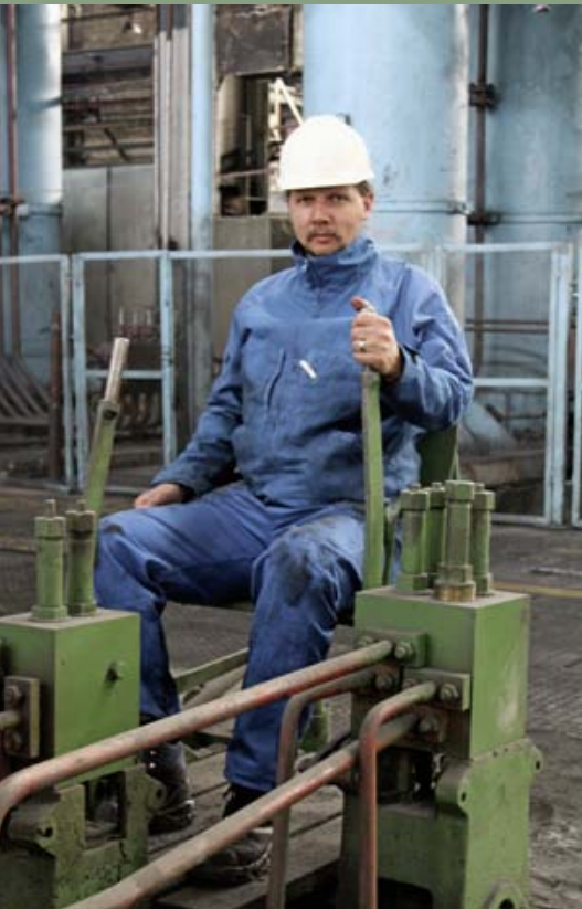
Press control prior to upgrade
